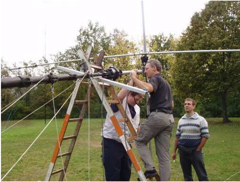
HB3YNV HB9IAB HB9DVA installing the beam
